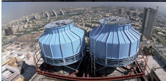
Cooling towers are usually installed on structures that already exist, so they need to be as lightweight as possible.
